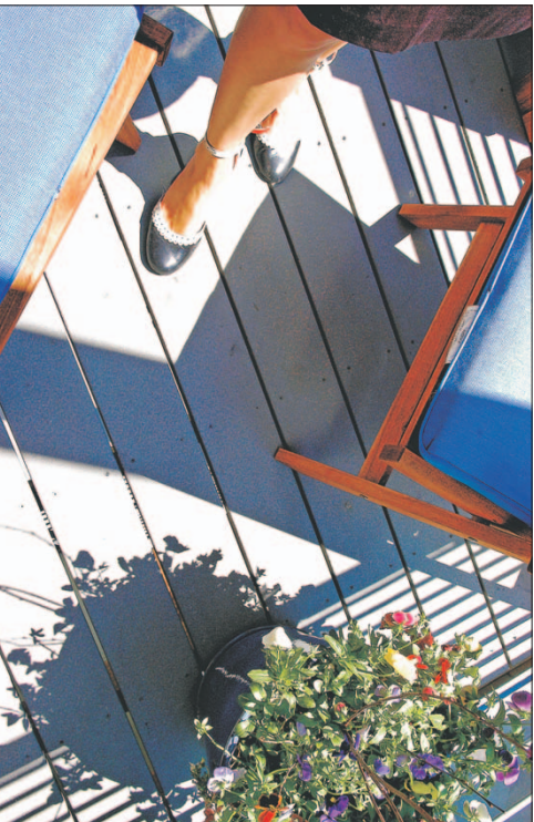
Photographs by Glen Stubbé/Star Tribune The outdoor decks at Midtown Lofts are constructed of Trex decking material, which is made of recycled plastic and waste wood and will not rot or deteriorate.
