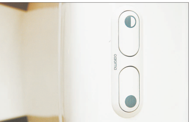
Dual-flush toilets conserve water by providing a low-volume, 1.6-gallon flush option (the button on the left).
